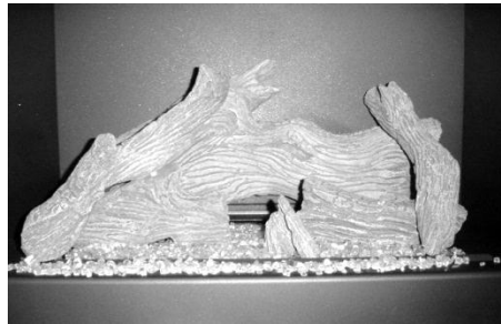
Figure 20: Completed Log Installation
