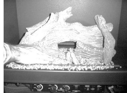
Figure 19: Spreading Crushed Glass
